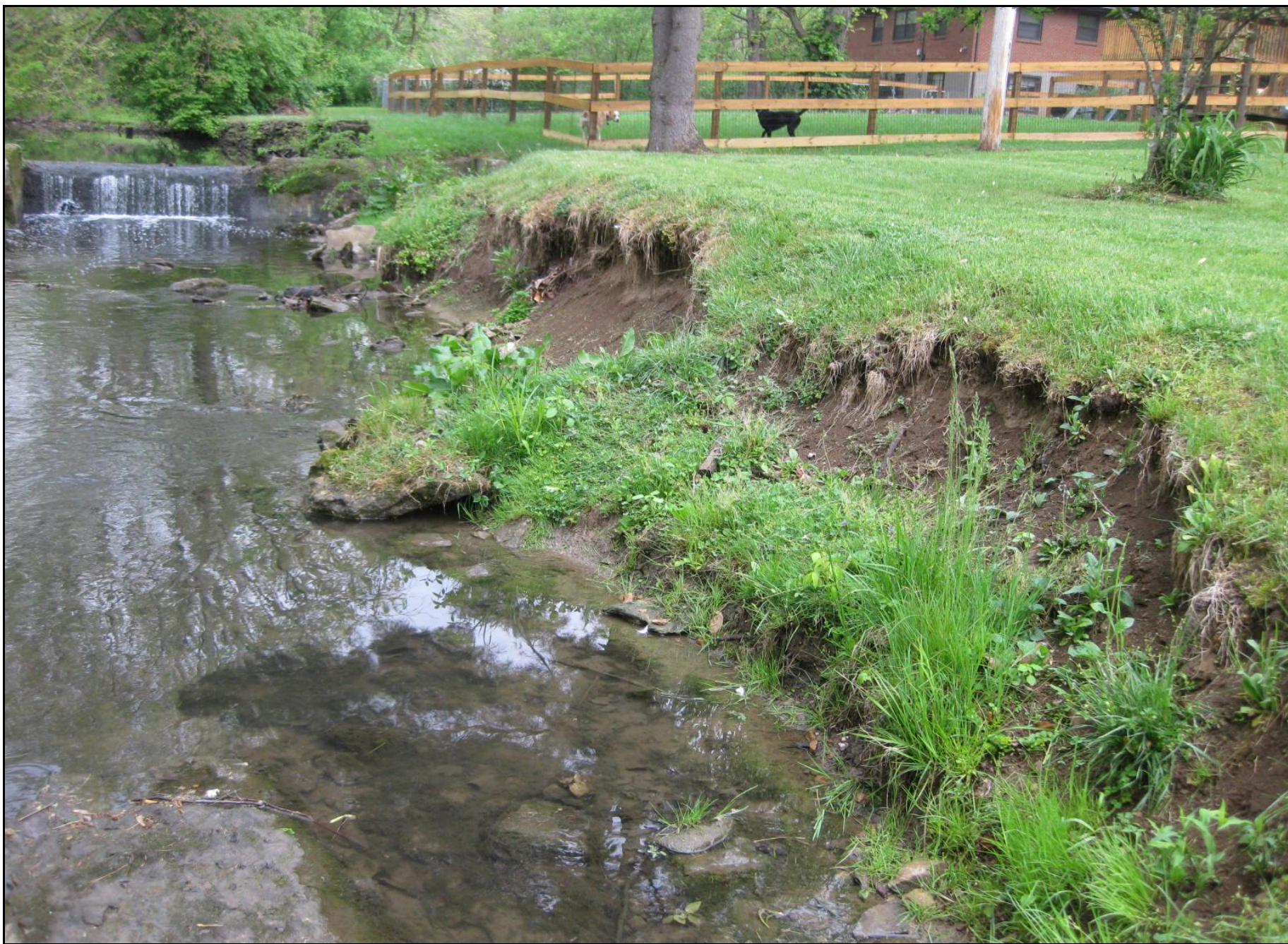
Eroding bank below dam, just upstream of public greenway; 2010 Apr 23.
