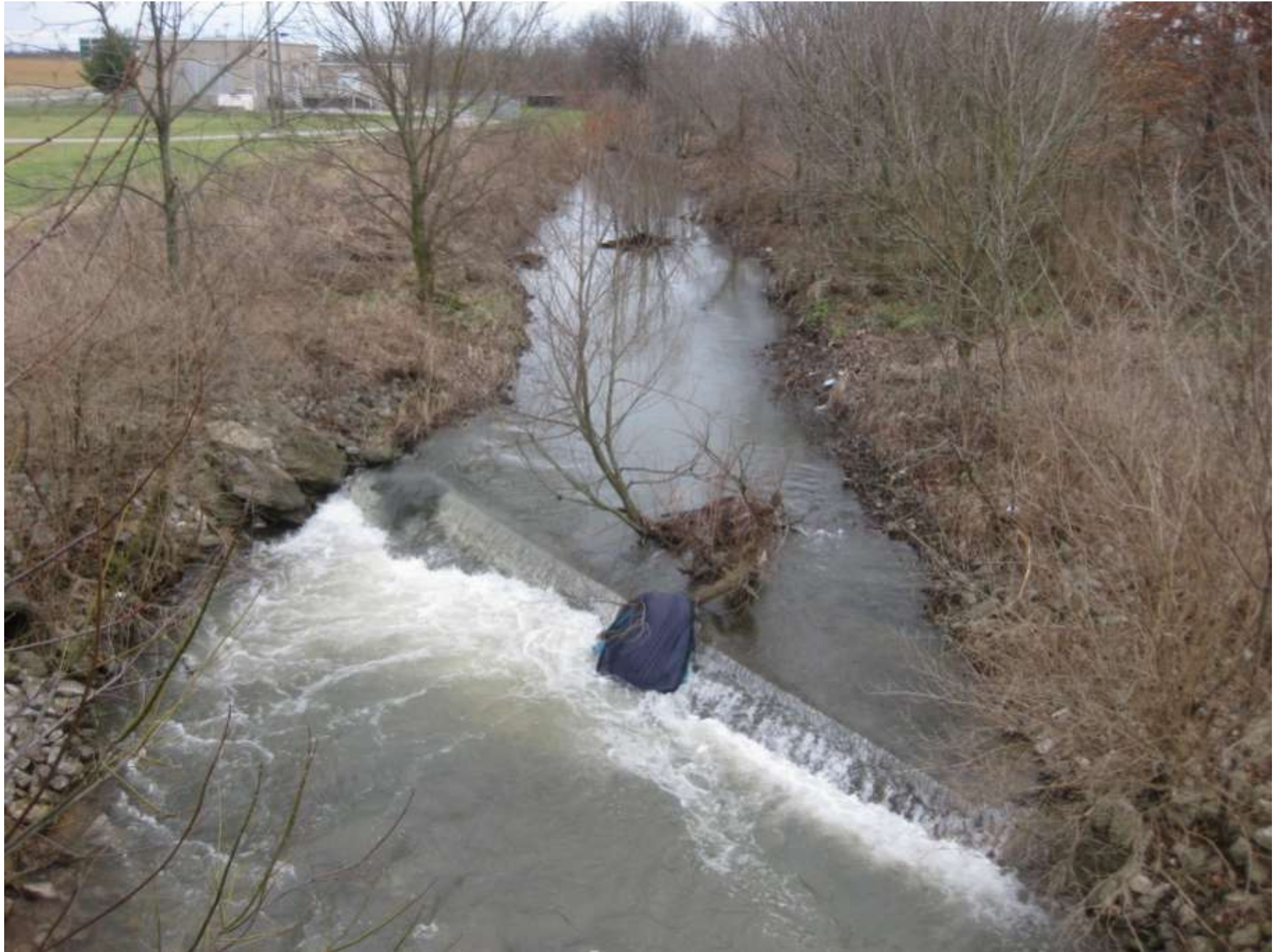
65: sewer line crossing creek just south of Legacy Trail bridge.
