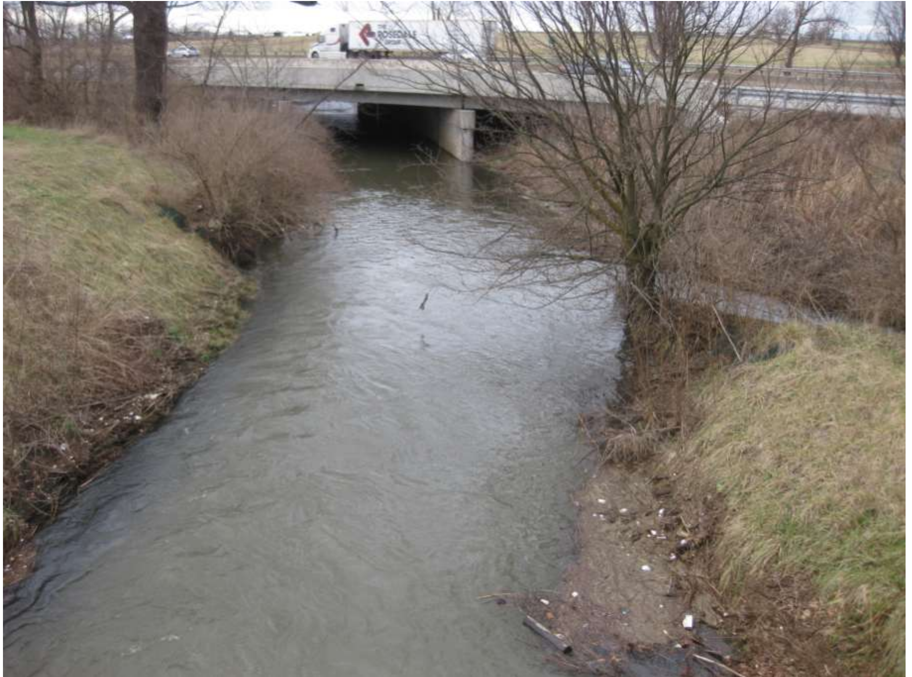
67: bridge under Interstates 64 and 75 (combined); junction with small tributary from east.
